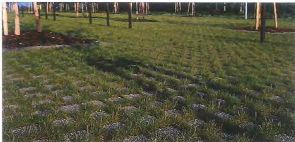
Illustration pavés perméable joints gravillons
